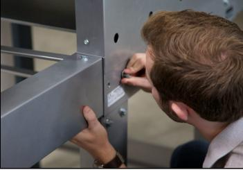
2. Insert a washer and leg bolt into one of the holes that connect the base and the arm.
