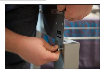
7. With the holes of the base and the leg aligned, insert a washer and hex bolt into the outer hole.
