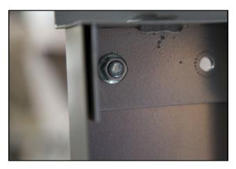
8. Tighten a lock nut onto the other side of the bolt, which faces inside the dryer. Only hand tighten it.
