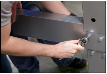
4. Using a wrench for the inside nut and a socket for the outside bolt, tighten the nut and bolt to hold in place. Tighten the other three bolts and nuts, leaving them loose enough to adjust for leveling.
